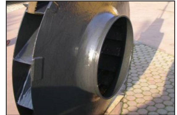
Completed application to 1600 mm fan
