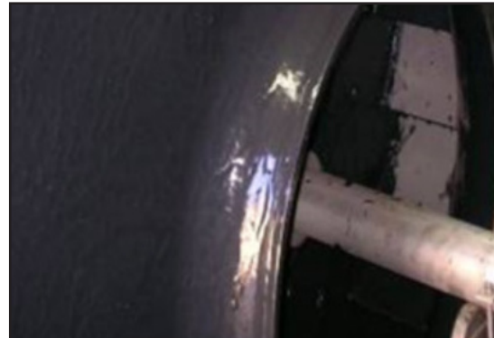
Fan being coated
